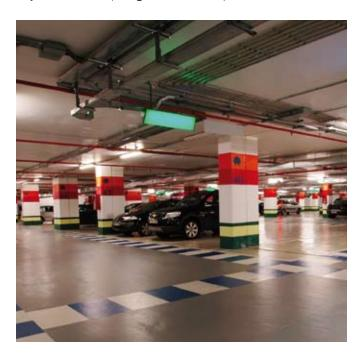
In jet ventilation, we use a completely different philosophy. Here, a small quantity of air is sucked into a fan and then ejected at high velocity. When this air hits the air in front of the fan, it thrusts it forwards while at the same time drawing the surrounding air along with it.
